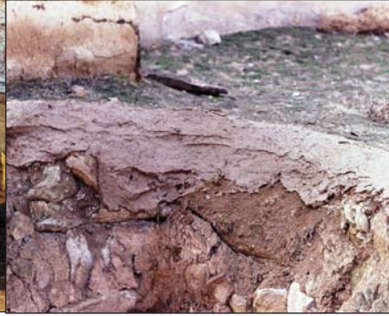
Figure 14. Contemporary use of mud plaster (clay) for maintenance. Photo by Uğur Tuztaşı 2010.
