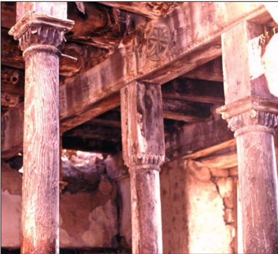
Figure 15. Hatipoğulları village room, wooden posts and detail relief. Photo by Uğur Tuztaşı 2010.
