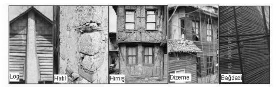
Figure 1. Types of wooden structures
