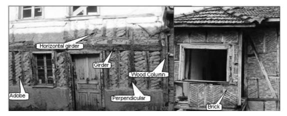
Figure 2. Details of a himis structure
