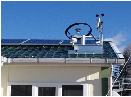
(a) Placement of measuring sensors.
