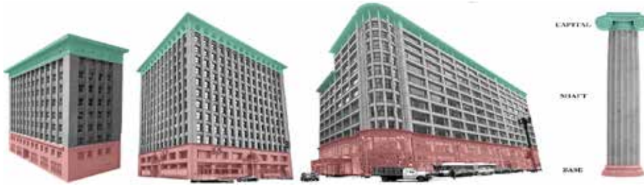
Figure 6: Façade composition of Sullivan's buildings: Wainwright Building, Guaranty Building, and Carson, Pirie, Scott, and Company Building.
